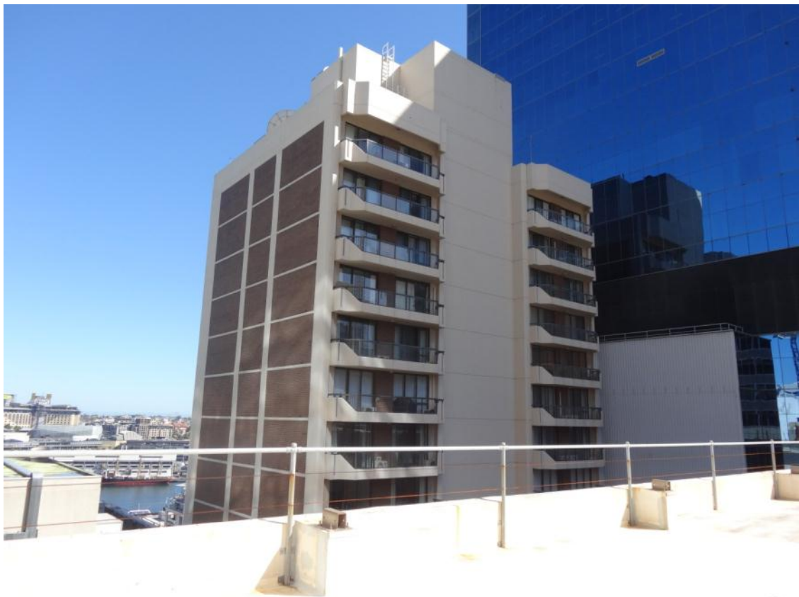
Figure 9: View from roof of existing building towards residential apartment building fronting Sussex Street
