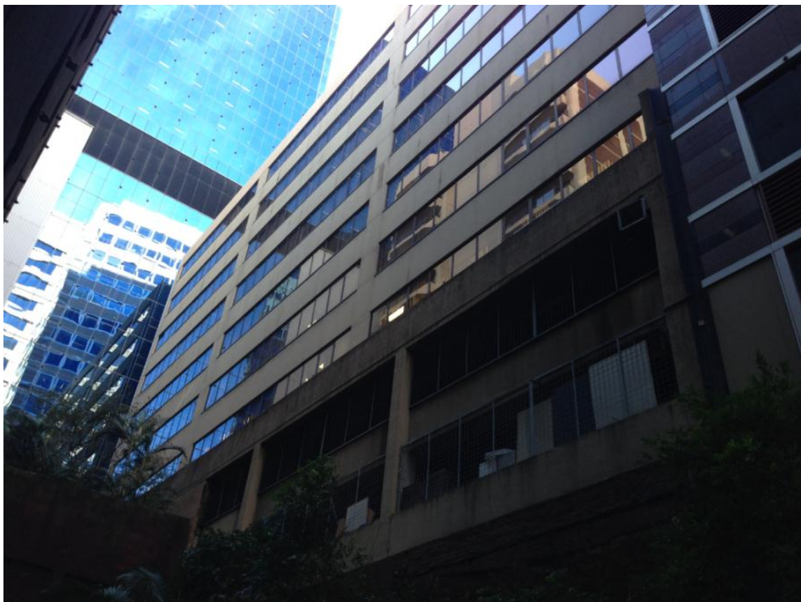
Figure 5: The upper levels of the rear of the existing building.
